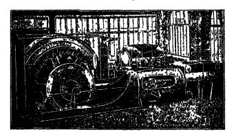
Illustration of 32" and 53" x 66" stroke; scroll and flat drum 12' to 16' diameter. Winding Engine for English Colliery. 1,650 ft. depth of shaft. Maximum duty, 2,900 tons of coal to be hoisted in 8 hours. Speed in shaft, 3,000 feet per minute,
